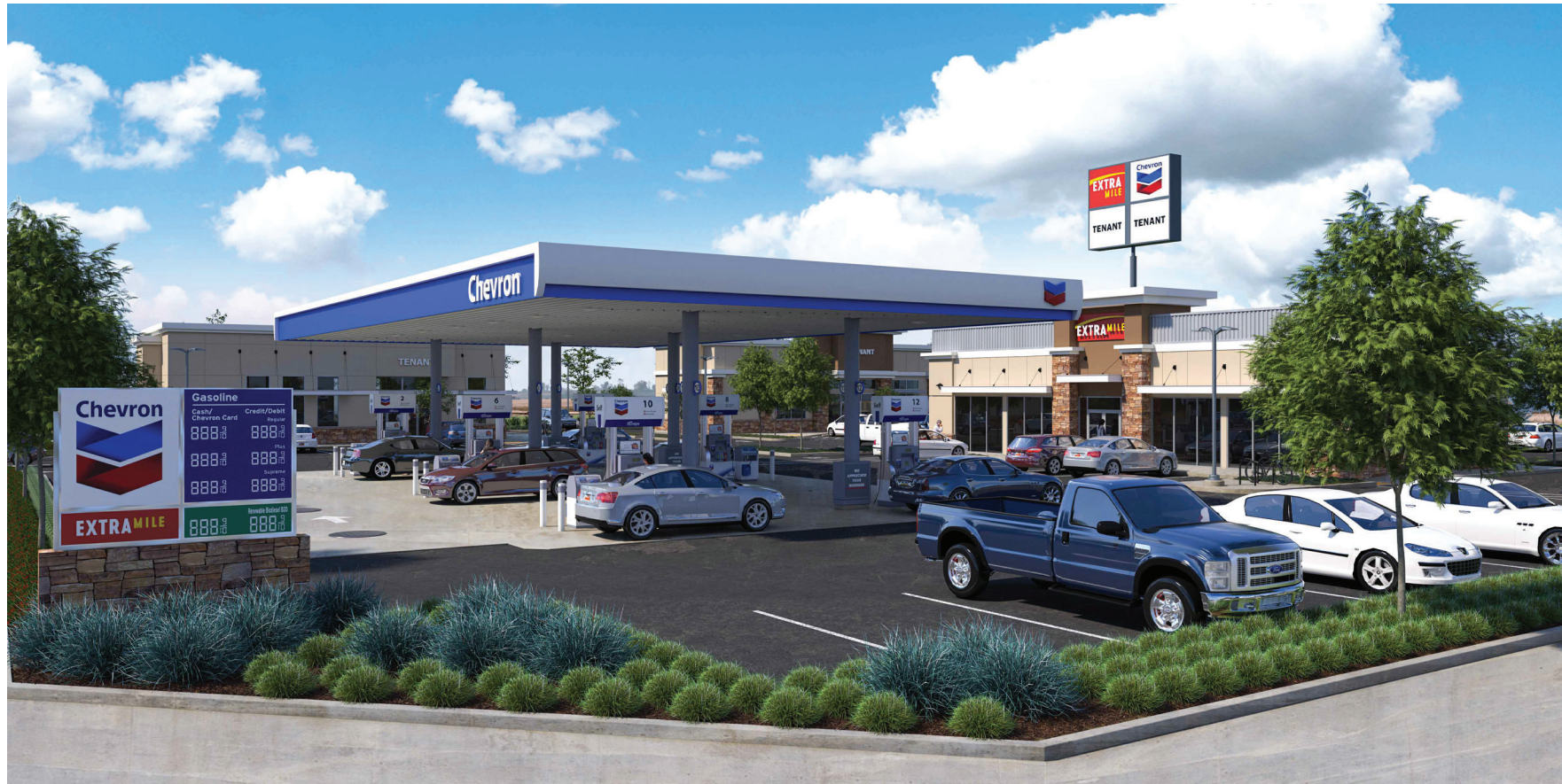
VIEW FROM ARCH ROAD and KINGSLEY ROAD CORNER
