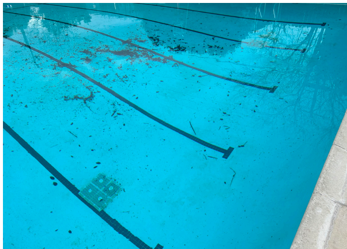
Image 25: Main Drain Cover in Swimming Pool
