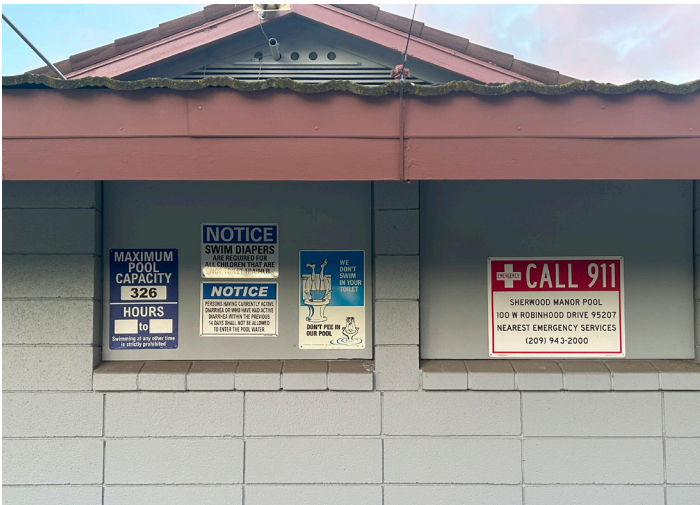
Image 9: Missing CPR Sign
