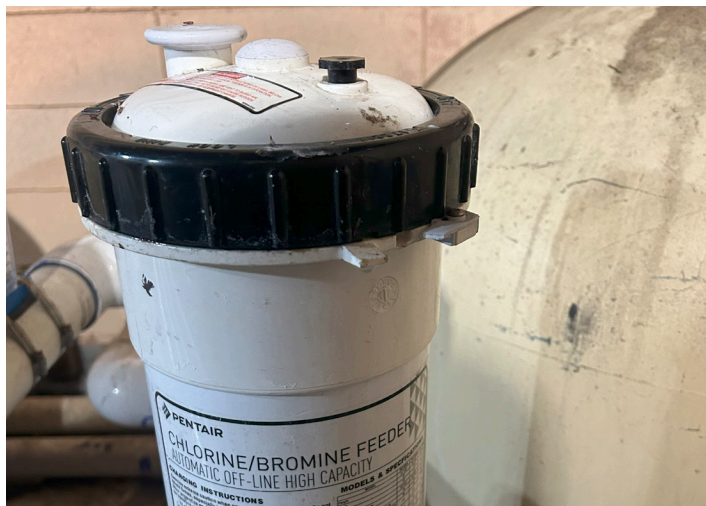
Image 1: Wading Pool Chlorine Tablet Feeder
