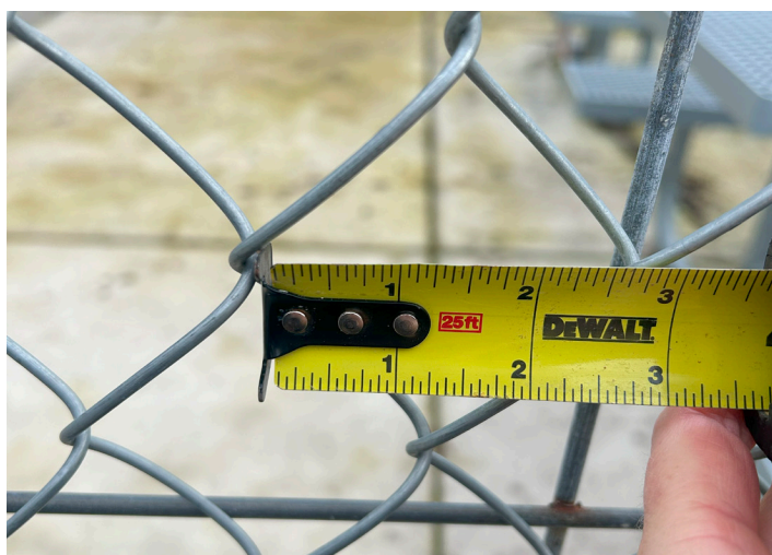
Image 17: Chain Link With Wide Opening
