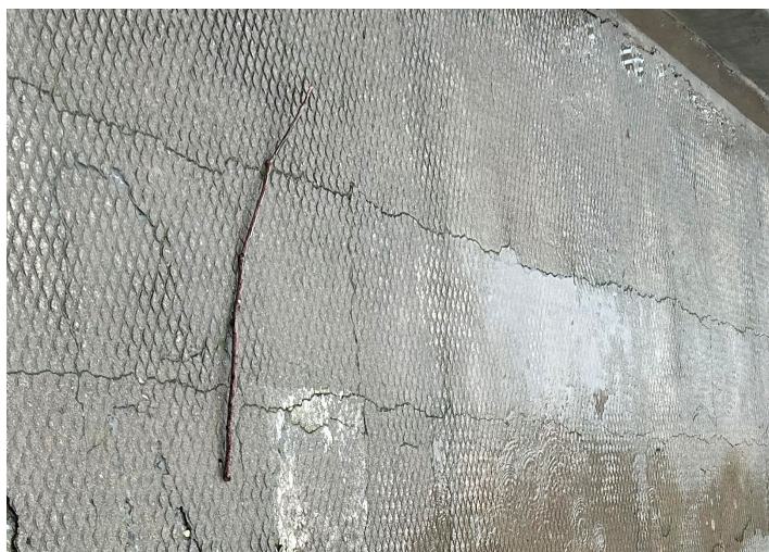
Image 48: Failing Deck
