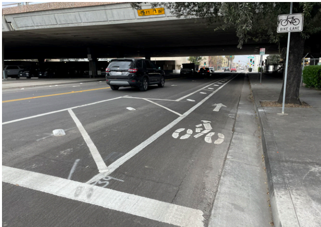
SR-4 underpass on California Street
