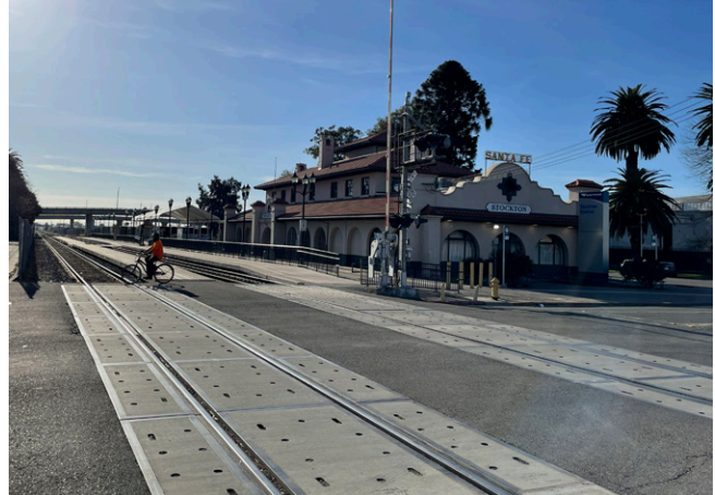
BNSF Tracks at San Joaquin Street Station
