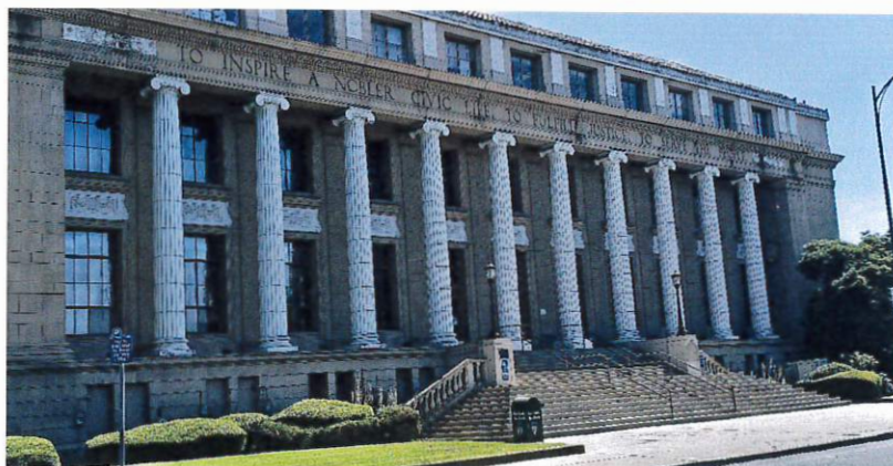
Front of Stockton City Hall (Photo by: Civil Grand Jury)
