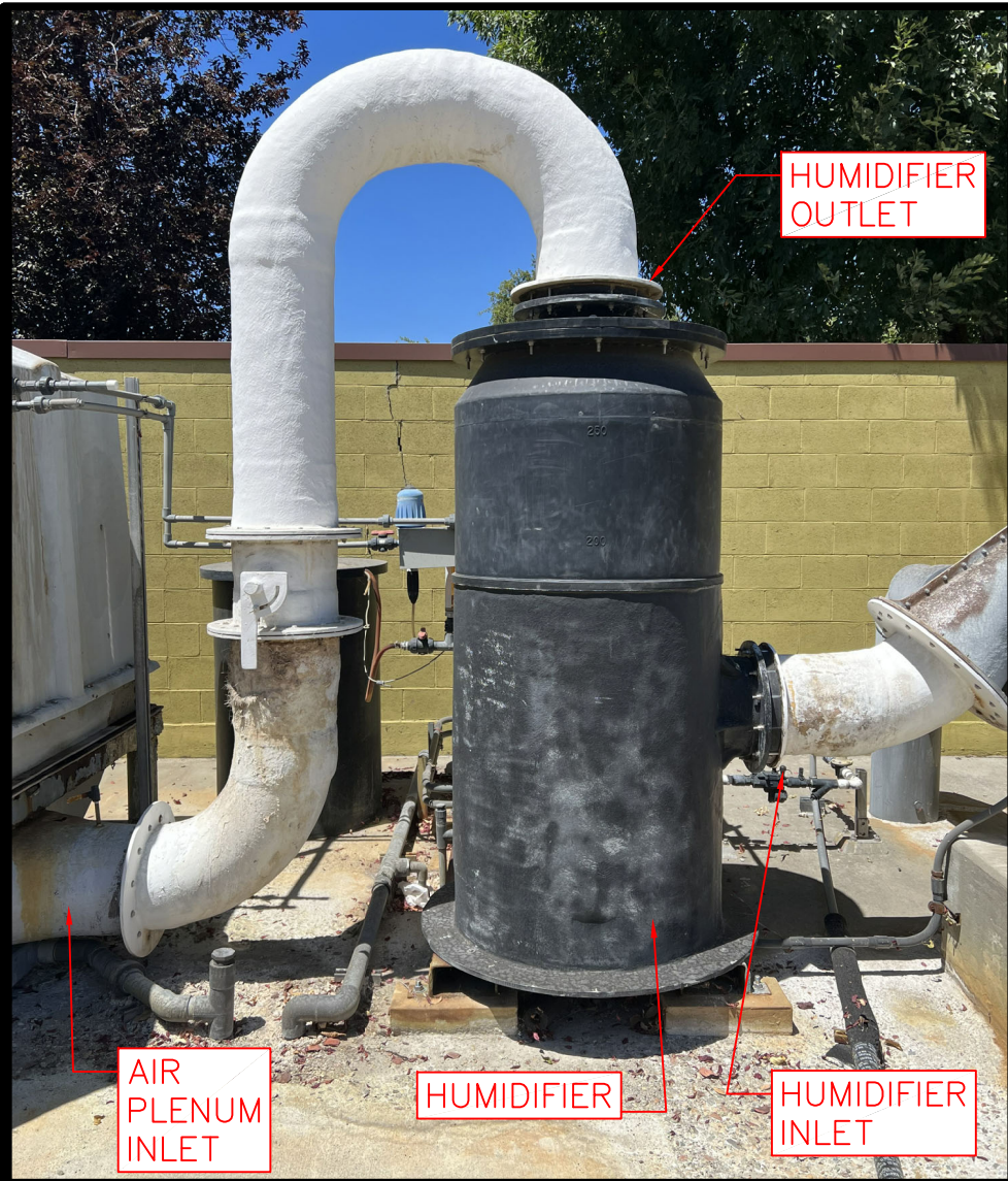
PHOTO 2 - EXISTING HUMIDIFIER
