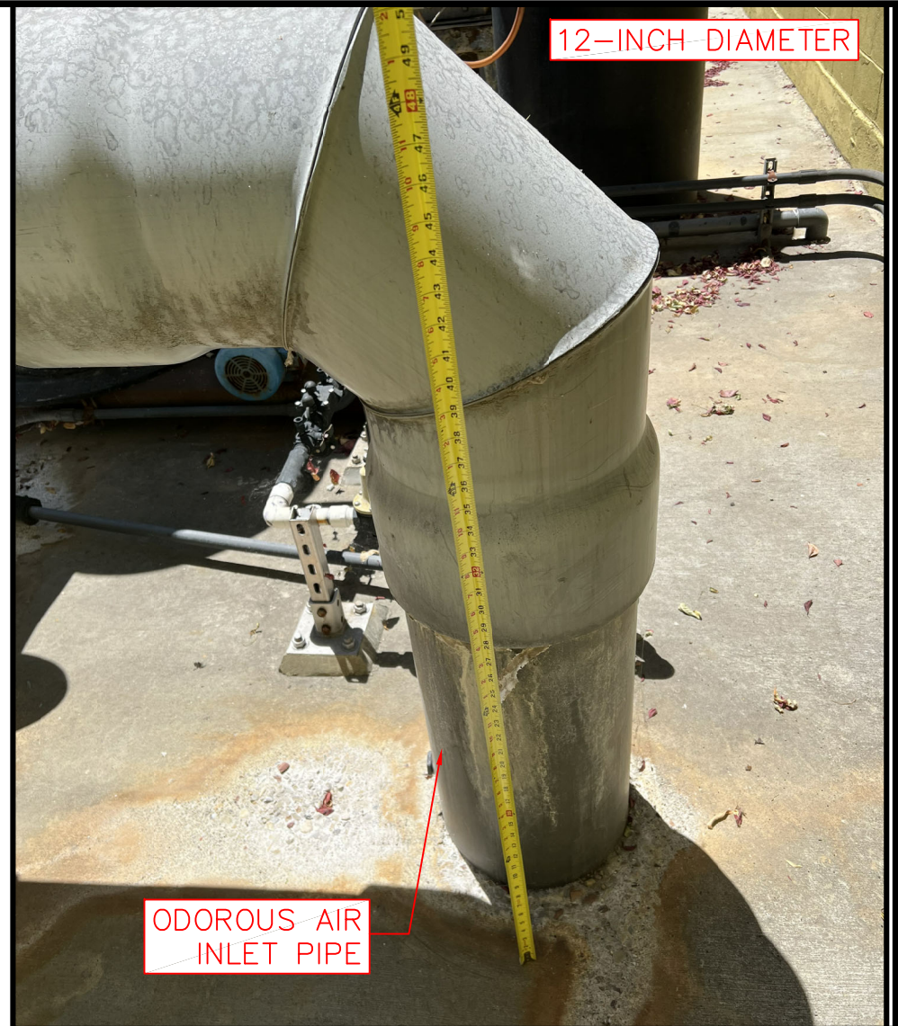
PHOTO 7 - EXISTING INLET PIPE
