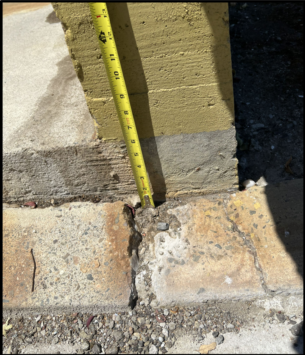
PHOTO 10 - EXISTING CONCRETE PAD
