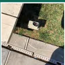
Junction box broken and submerged in water.
