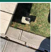
Junction box broken and submerged in water.
