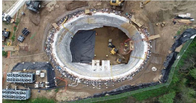
Jeff was the CM and Matt the inspector on this excavation using soil freezing - SRWA
