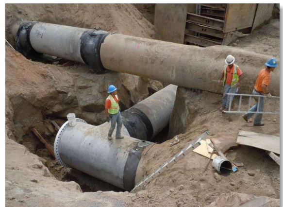
72-inch pipeline at SJWD WTP
