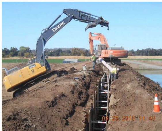
Pipeline installation in the berm between percolation basins – Ione WWTP
