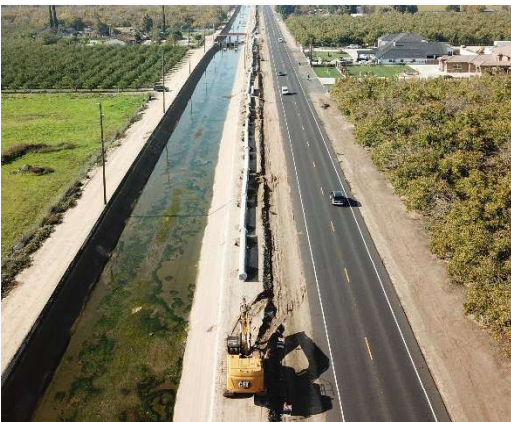
Jeff was the CM and Matt the inspector on 7 miles of 42" steel pipe - SRWA
