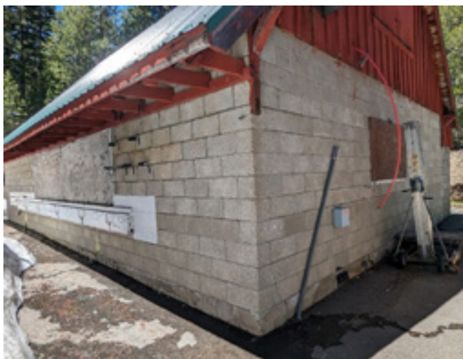
Figure 10: Exterior Southeast Corner of Kitchen
