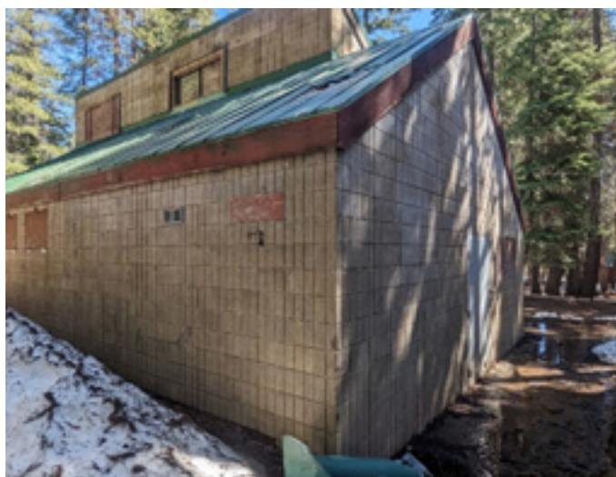
Figure 6: Restroom and Showers West Exterior View
