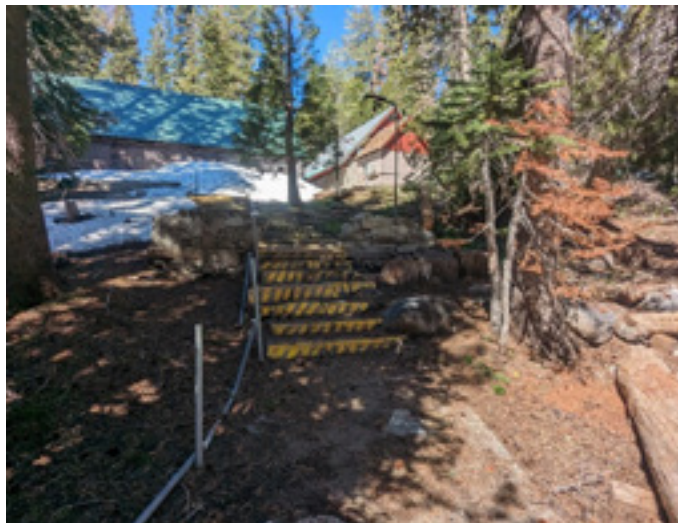
Figure 5: Cabin P Exterior with Manager's Office at Left
