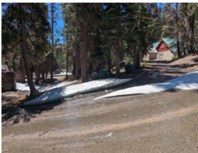
Figure 1: Lodge Approach Roadway Cross Slope
