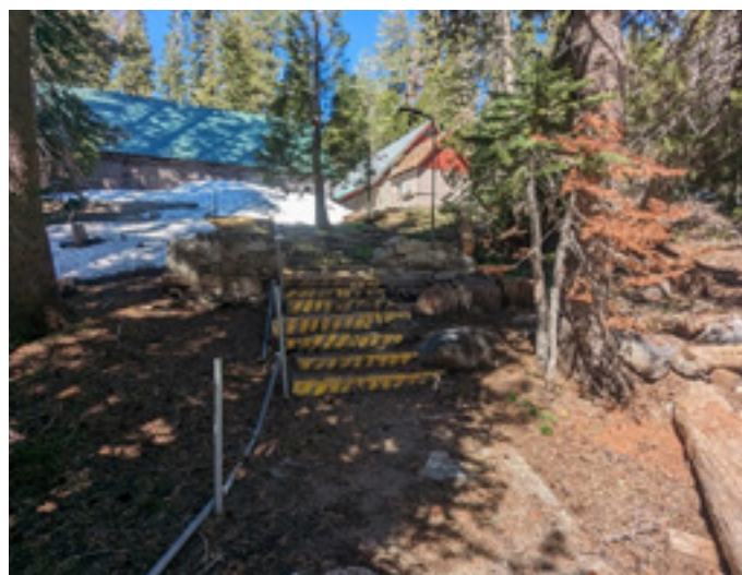
Figure 2: Exterior Stairs East of Lodge Shown on Left. Fire Pit is On Right Side of View
