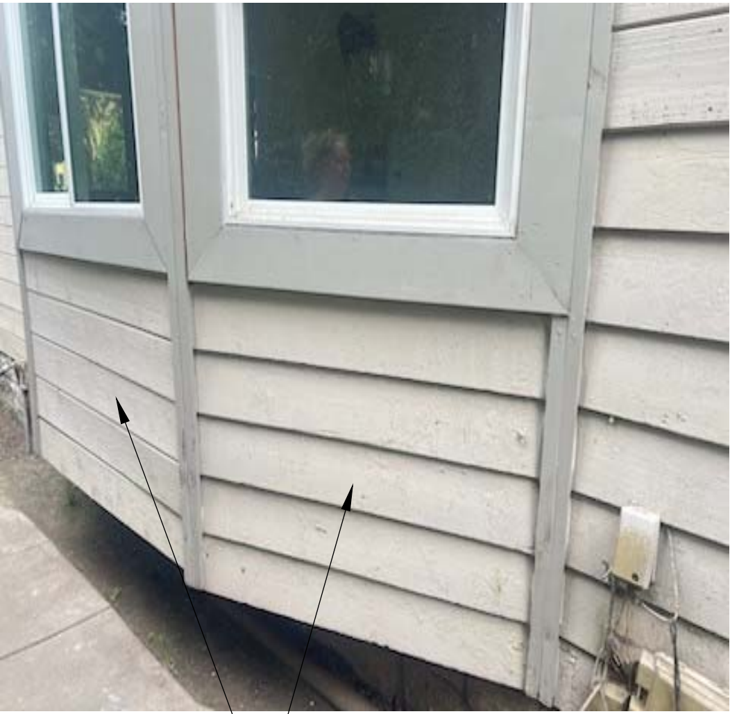
Siding Repaired w/ Matching Line Pattern
