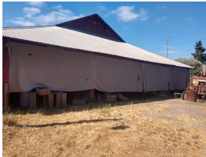
Figure 11 – View of barn facing south.
