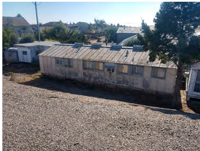
Figure 14 – View abandoned “barracks” structure.
