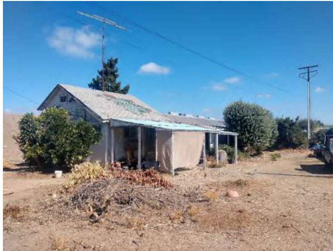
Figure 15 – View of abandoned house structure facing northwest.
