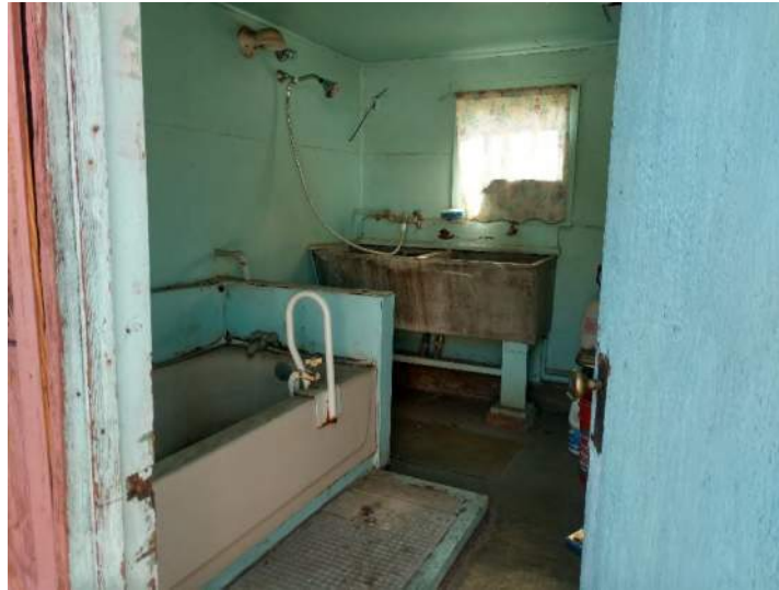
Figure 9 – Inside view of bath house.
