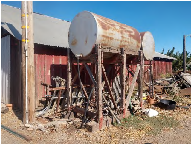
Figure 3 – View of two ASTs adjacent barn.
