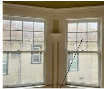
Existing Window Grid Pattern
