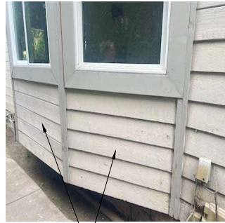
Siding Repaired w/ Matching Line Pattern
