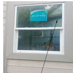
All New Windows To Have A Vinyl Grid Pattern Added To Match Existing Windows As Close As Possible
