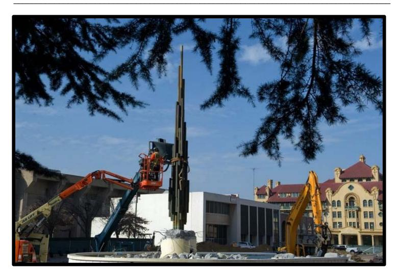
The spire located in the Hunter Square fountain being removed in preparation of the demolition work associated with reconstructing the San Joaquin County courthouse.
