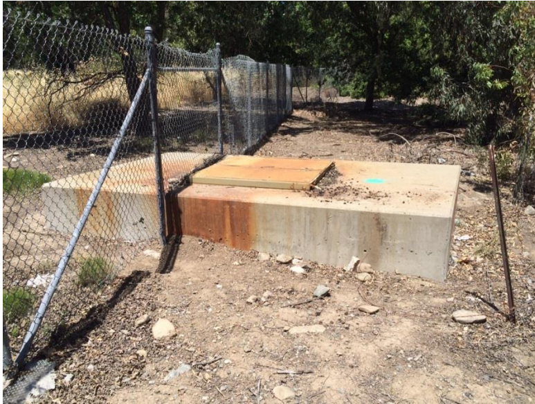
Van Buskirk Inlet Vault- Corroded Cover
