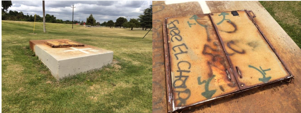
Van Buskirk Outlet Vault-Corroded Cover
