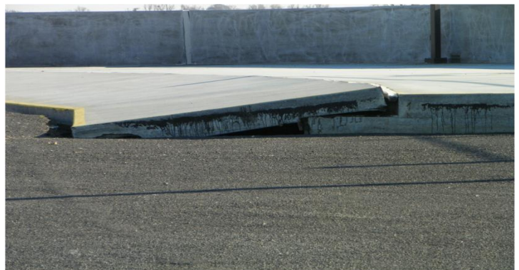
A concrete slab has shifted due to soil settling at the IPS.
