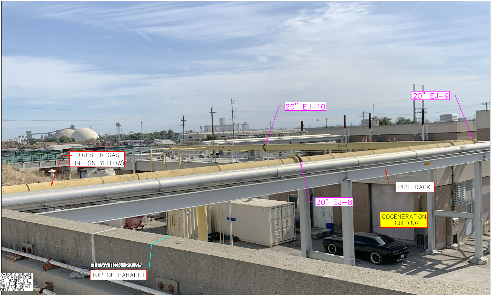
PHOTO 17 – NORTH-EAST VIEW FROM SLUDGE BUILDING ROOF
