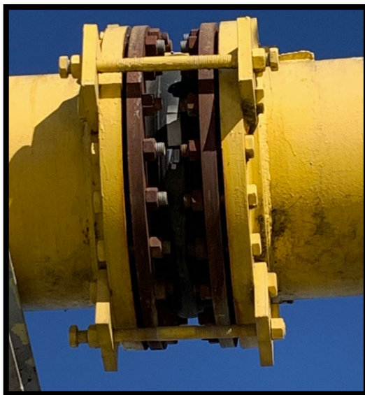
Figure 2. Welded Pipe-Flange Connection
